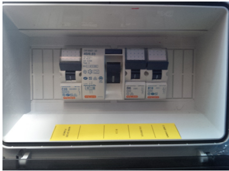
220V shore power switchbox
