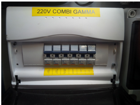
220V combi Gamma switchboard
