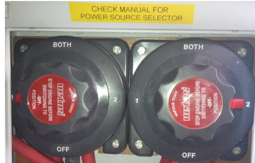
Start battery selector switches
