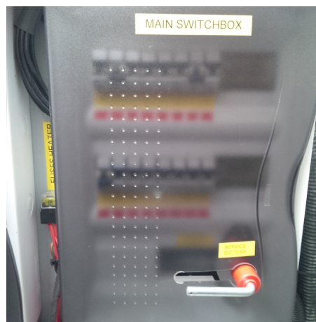
Service battery switch
