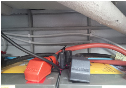
Active corrosion fuses (2x 1Amp)
