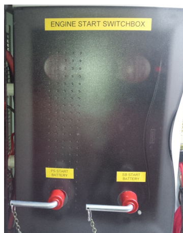
Start battery switches
