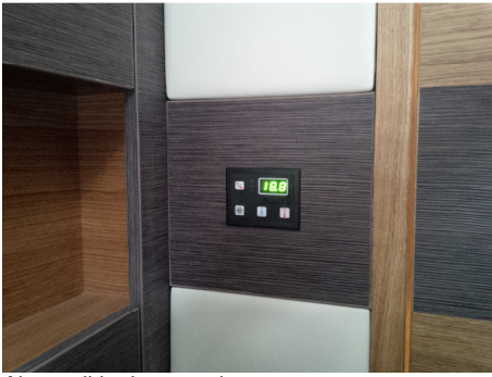
Air conditioning panel
